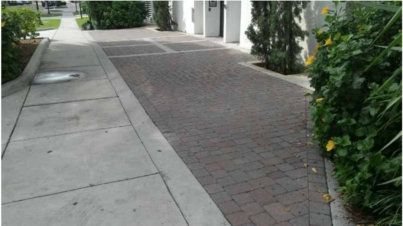
Entry Drive - Eola Drive
