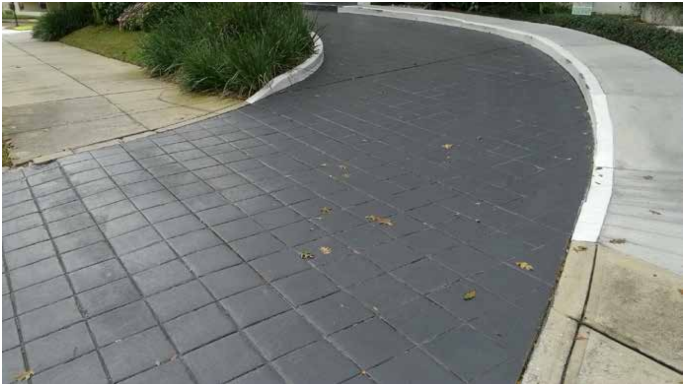
Entry Drive - Central
