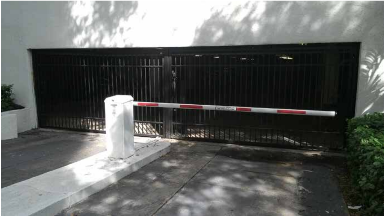
Garage Access - P1
